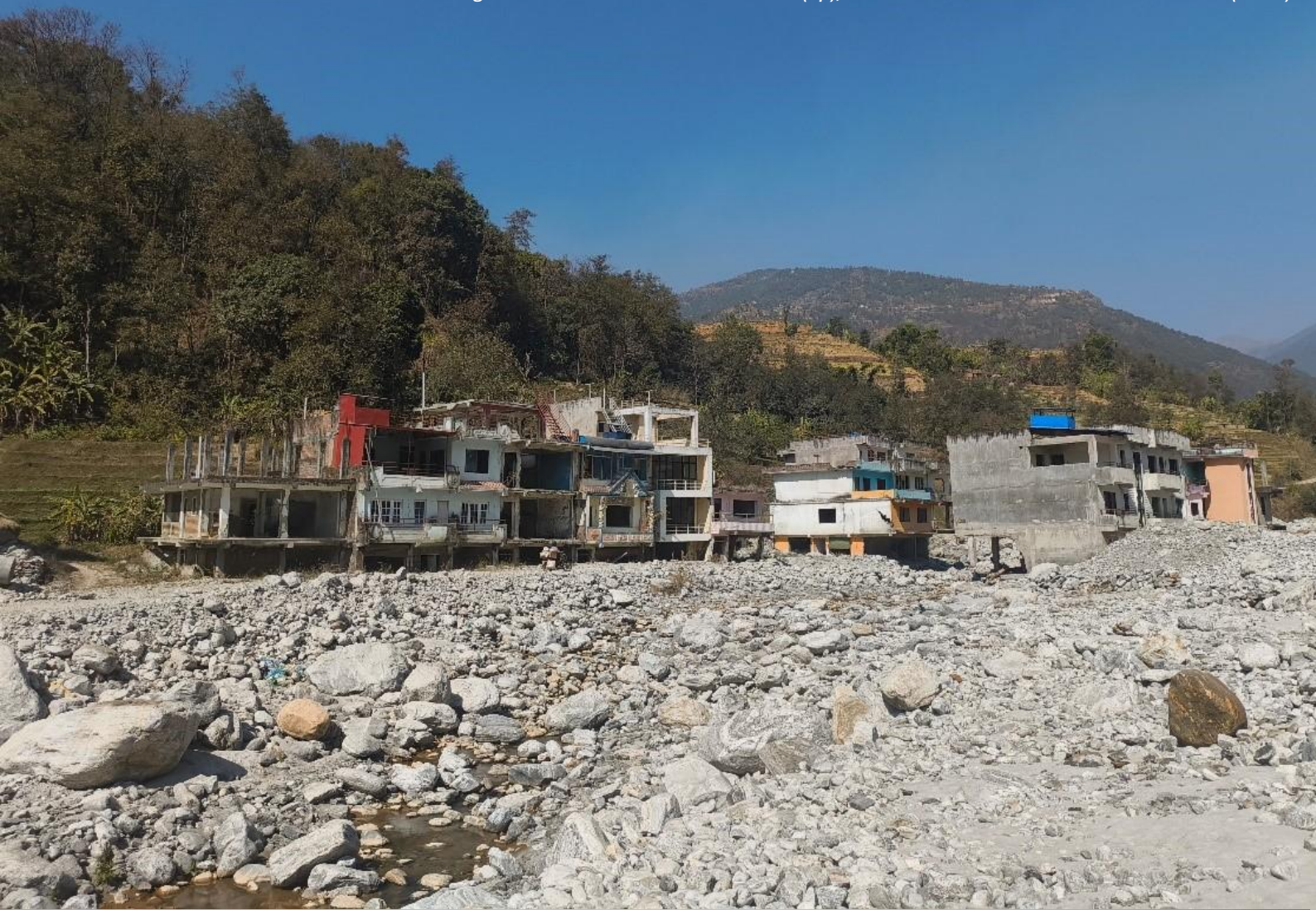
Figure 17: Chanaute Bazaar settlement (up), debris filled interiors of the affected houses (down)
